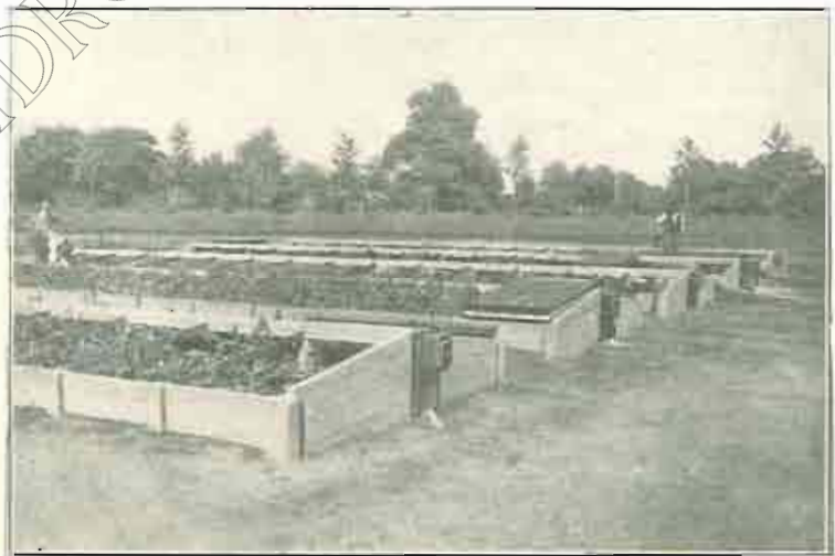
CAJONERAS TERMOELECTRICAS SIEMENS
